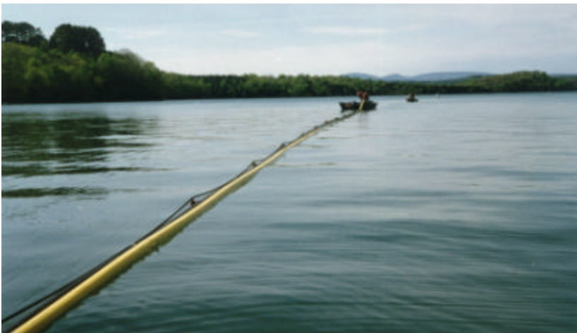
Figure 3: Line Diffuser Deployment Without Divers
