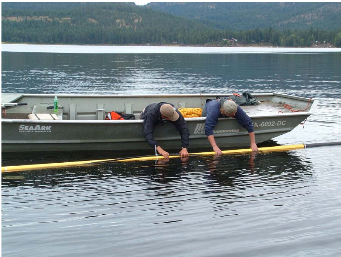
Figure 47. Checking oxygenation system before submerging
